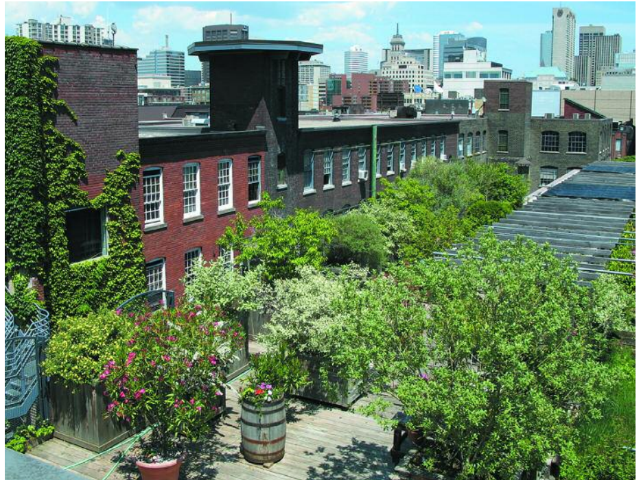
The roof of Toronto's 401 Richmond building has a 6,500-square-foot cedar deck with flowers, vines, and shrubbery; a 2,600-square-foot garden; and a 40-foot greenhouse
